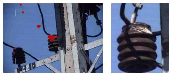
Fig. 9, 10. Corona discharge and its effects.
